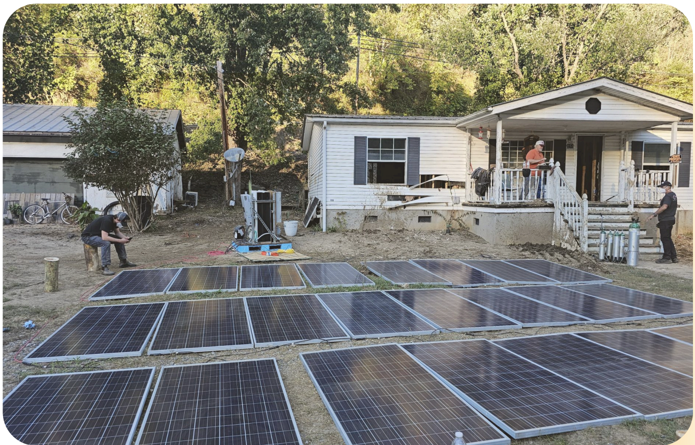
Footprint Project installs solar panels in the aftermath of Hurricane Helene.
