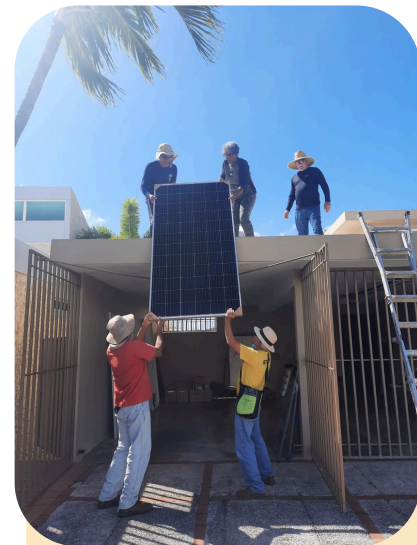
Solar system installation workshop led by AMANESER in Barrio Candelerero, Humacao.
